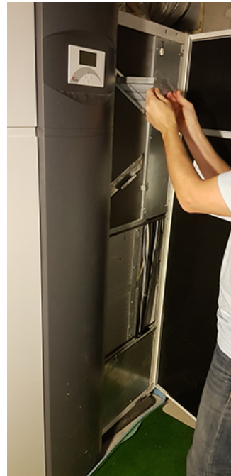
Replacing the filter cassette in the system
