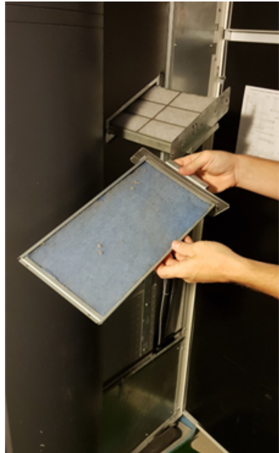
Removing the dirty filter mat
