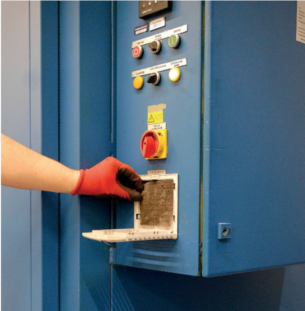
Removing the dirty filter mat
